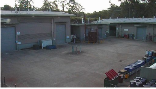
Figure 2: The test environment at daytime. The reflective beacons used in the laser beacon localisation system can be seen as white tape attached to bollards. The environment measures approximately 50m by 35m.
